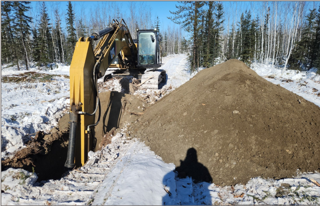
Photo 3: Borrow Source BS899, Testpit Excavating Excavating for Testpit TP25-BS899-03 (Photo Date: March 26, 2025)
