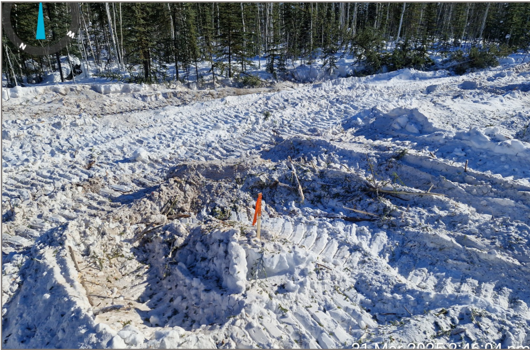
Photo 2: Borrow Source BS899, Site Access Clearing Site access clearing completed for Testpit TP25-BS899-03 (Photo Date: March 21, 2025)
