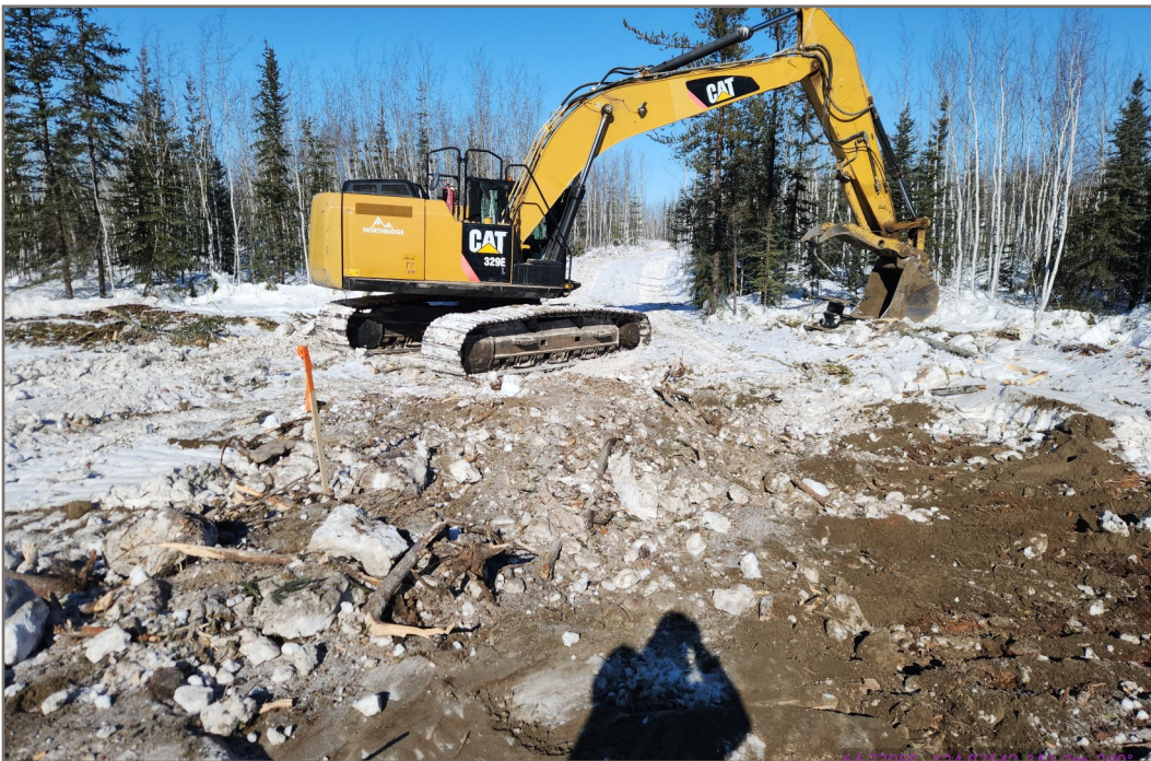
Photo 4: Borrow Source BS899, Testpit Excavating Completed and backfilled Testpit TP25-BS899-03 (Photo Date: March 26, 2025)
