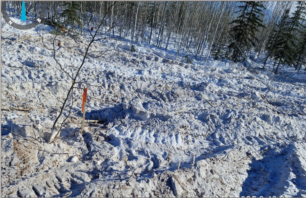
Photo 1: Borrow Source BS899, Site Access Clearing Site access clearing completed for Testpit TP25-BS899-02 (Photo Date: March 21, 2025)
