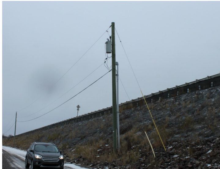
Figure 3-5: Utility Line on North Part of Deh Cho Bridge
