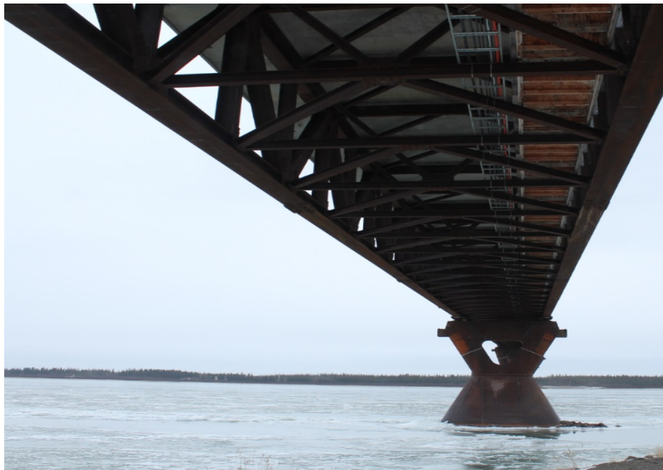
Figure 3-3: Deh Cho Bridge for Mackenzie River Crossing
