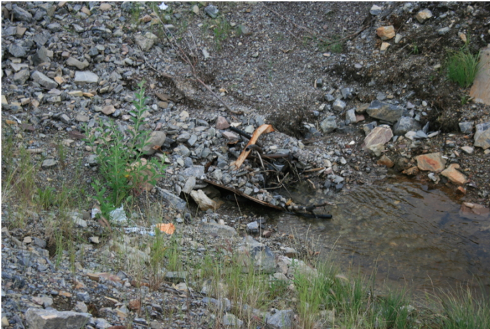
Photo 13. Outlet for culvert under Taxiway B (July 2015).
