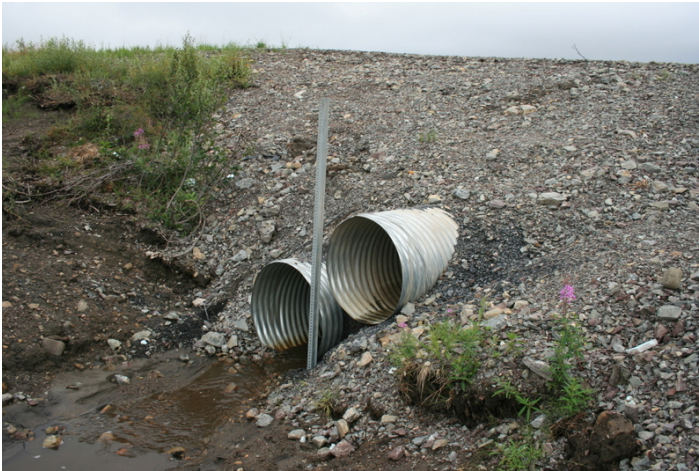
Photo 7. Double culvert installed under access road on east end of the runway (July 2015).
