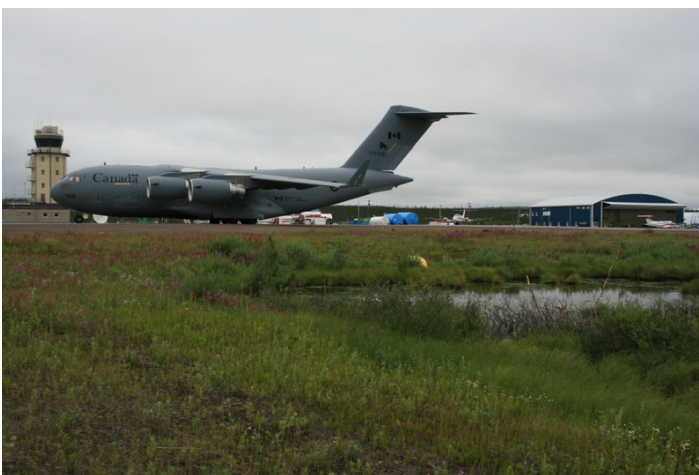
Photo 9. Water ponding in the infield between runway and Taxiways A, B and D (July 2015).
