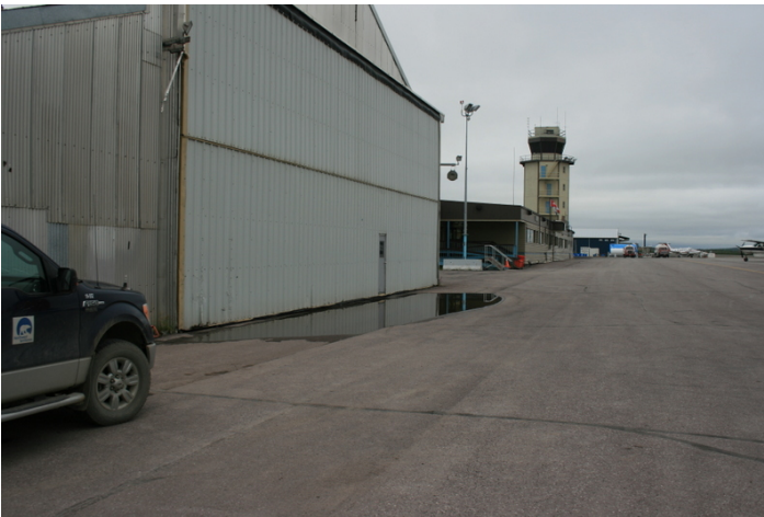
Photo 17. Water ponding next to hangar building looking towards air terminal building (July 2015).
