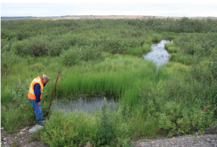
Photo 12. Inlet for culvert under Taxiway B (July 2015).
