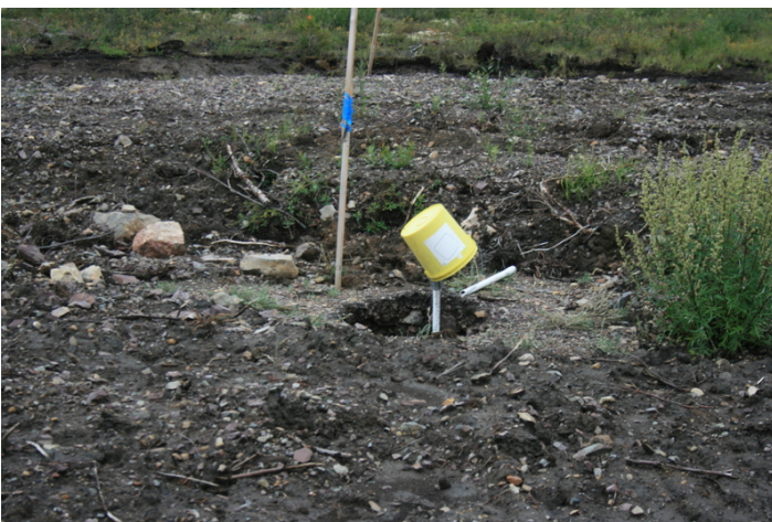
Photo 21. Thermistor installation on east end of runway (July 2015).
