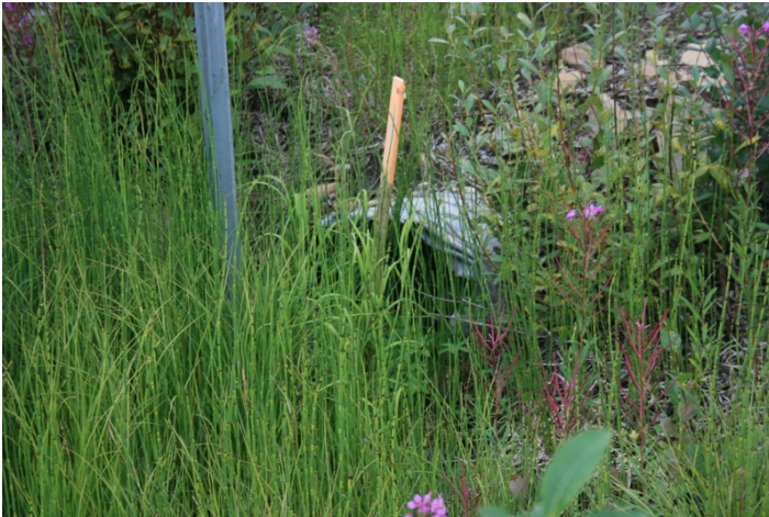
Photo 10. Inlet for culvert under Taxiway D (July 2015).
