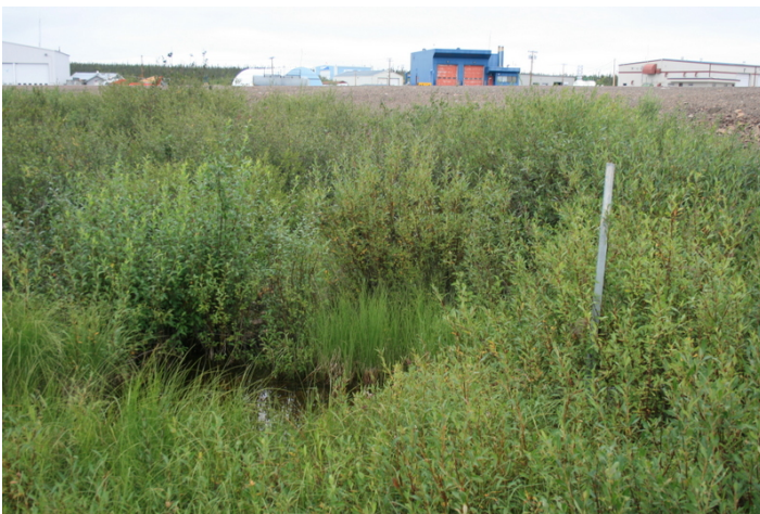
Photo 11. Outlet for culvert under Taxiway D (July 2015).
