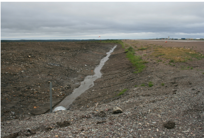
Photo 8. New diversion ditch on the south of runway (July 2015)
