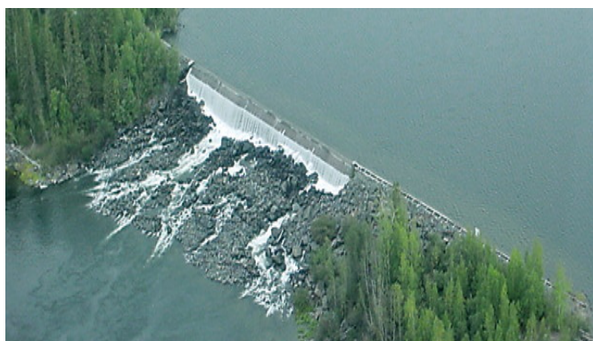
Figure 13: Bluefish Dam (Source: NWT Power Corp)
