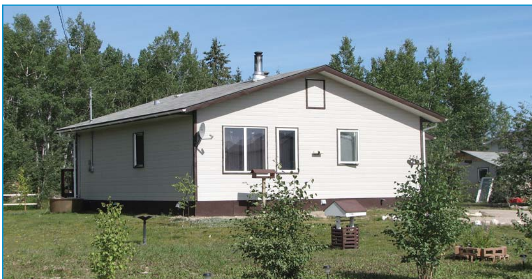
Fort Providence, NWTHC PHOTO
